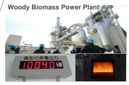
Power Generation Capacity: 10,000 kW (Annual Power Generation: Approx. 80,000 MWh) About 110,000 tons of fuel is used per year. In principle, only locally-sourced wood is used.
